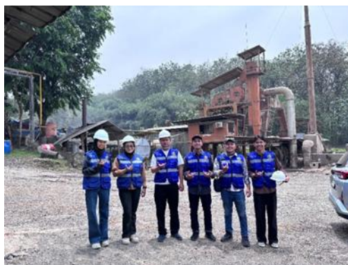
Gambar 4. 1 Asphalt Mixing Plant (AMP) PT. Deltamarga Adyatama Batang (Sumber: Dokumentasi Pribadi)
